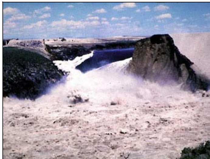
Teton Dam Disaster 1976, someone pulled the plug out.
